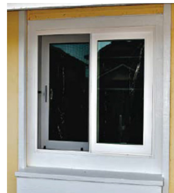
Figure 4-21. Impact-resistant glass installed in a window, which adds protection from strong winds and debris from hurricanes and tornadoes. (Source: Hawaii Sea Grant)
