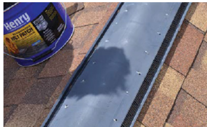
Figure 4-10. The ridge vent (on right) is applied over the roof ridge and is secured by doubling the nailing pattern. This strengthens the ridge vent and makes it less vulnerable to being blown off in a storm. (Source: Hawaii Sea Grant)
