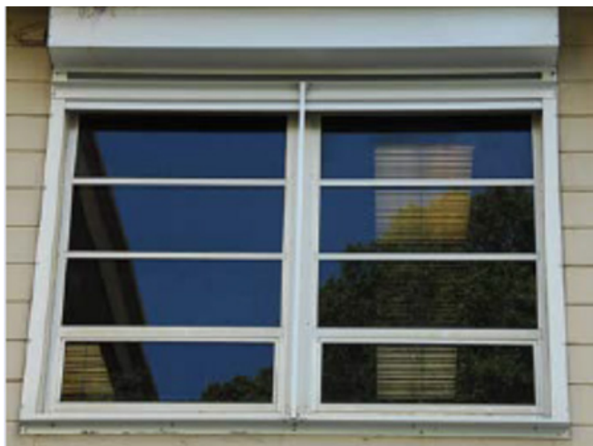
Figure 4-17. Roll-down shutters applied to a home. These can be deployed electronically or manually. (Source: Hawaii Sea Grant)
