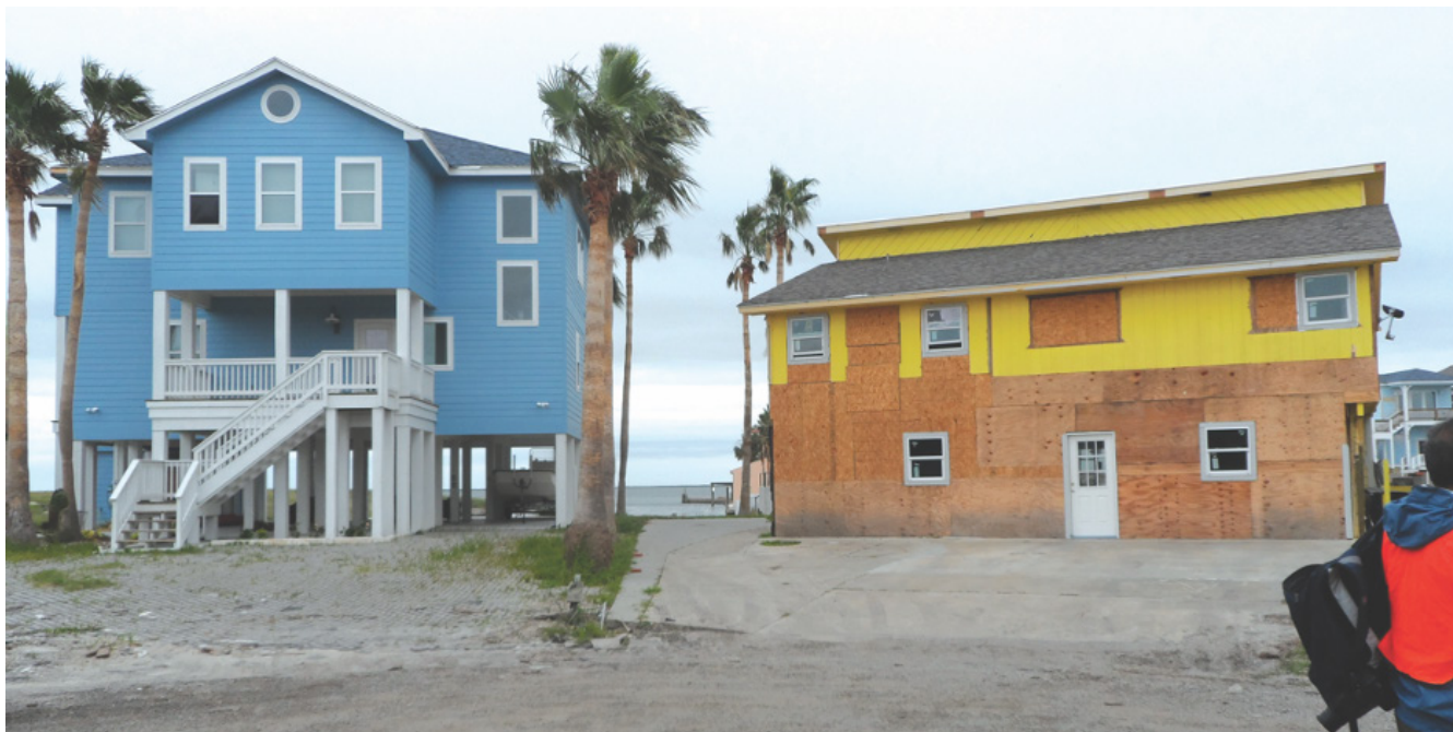
Figure 4-31. A beach house elevated (left) next to a beach house on the ground (right). (Source: Texas Sea Grant)
