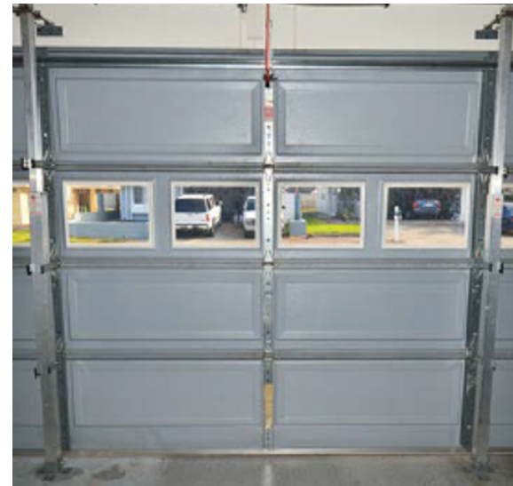
Figure 4-22. Vertical braces on the garage door run from the top and are connected to fasteners that are built in to the concrete floor. This strengthens the garage door during storms with high wind events. (Source: Hawaii Sea Grant)
