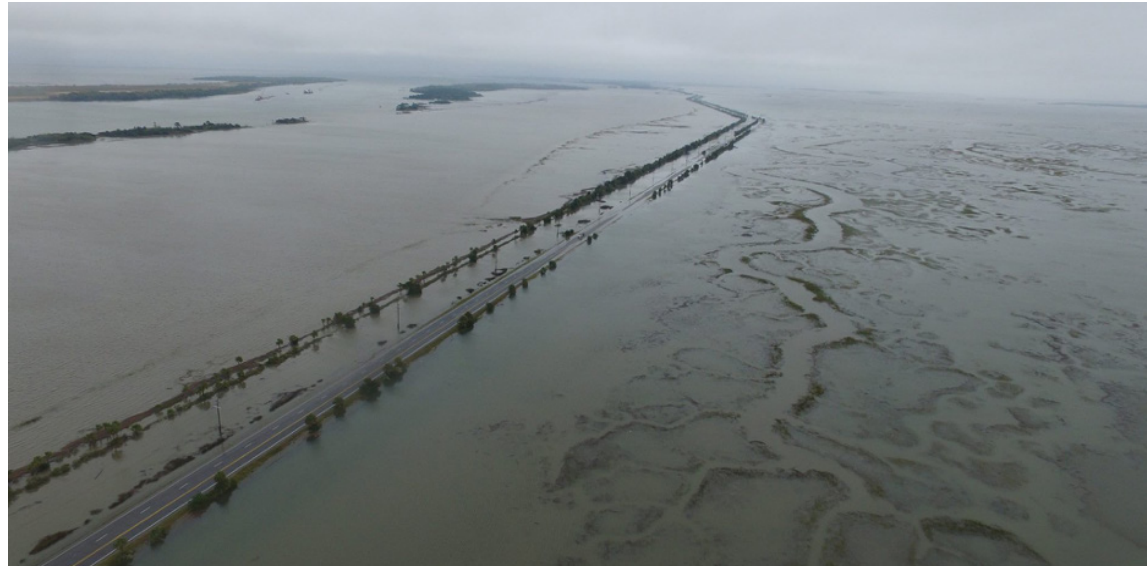
Figure 2-11. A picture of Highway 80 flooding towards Tybee Island. (Source: Sean Compton)
