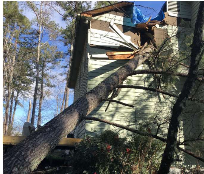
Figure 2-4. A photo of a fallen tree on a house in Paulding/Cobb County, Georgia, caused by a tornado and straight-line winds. (Source: National Weather Service)
